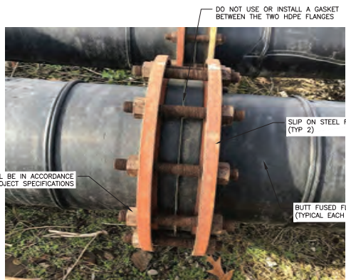
SLIP ON FLANGE CONNECTION 2 NOT TO SCALE 00C-09
