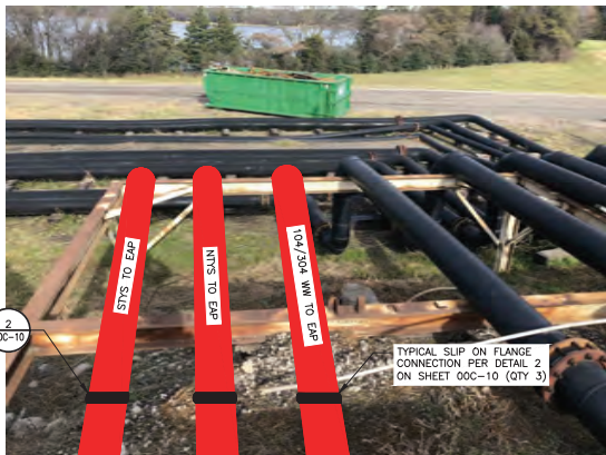
TERMINATION DETAIL C AT EXISTING PIPE RACK (C) 00C-09 NOT TO SCALE
